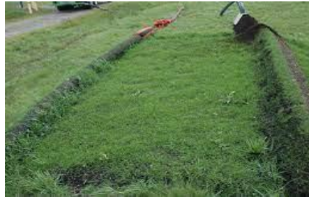
Figure 7. Erosion control in agricultural fields (photo: www.stancounty.com )
