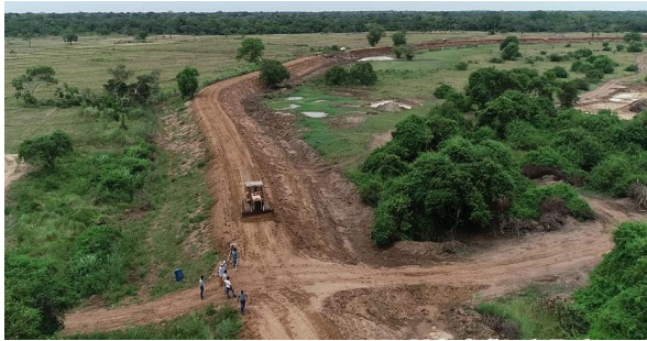
Figure 4. Agri-road construction (photo: CSIAP)
